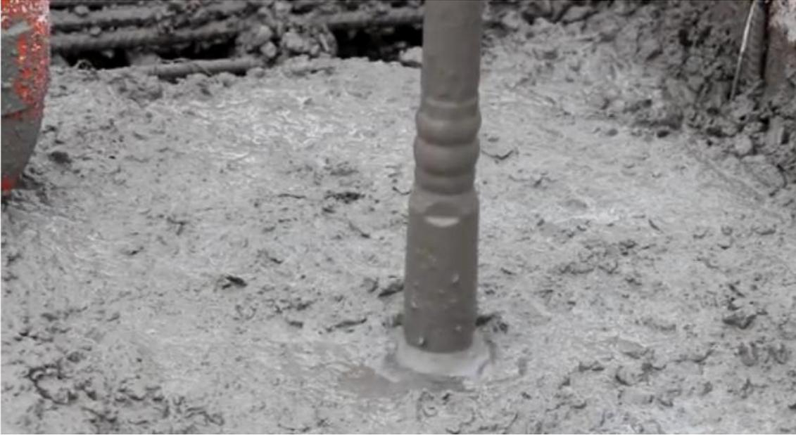
Remove the head slowly and smoothly allowing the hole to fill in behind it. Removing too quickly will leave behind a void in the concrete.
