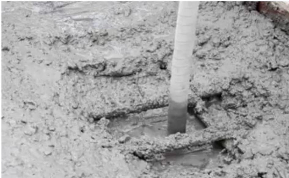
Avoid vibrating against the rebar. Keep a distance of at least 50mm or more.
