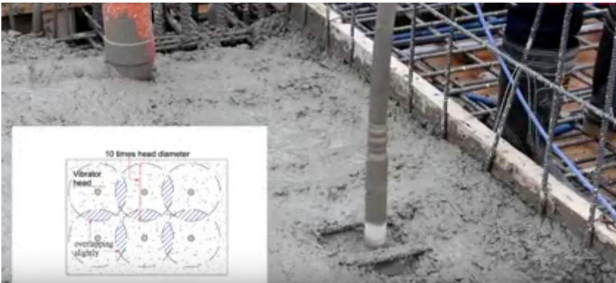
The area of effect is roughly ten times the head diameter and slightly more than the head's height. So for ideal compaction the head should be inserted at regular and slightly overlapping intervals.
