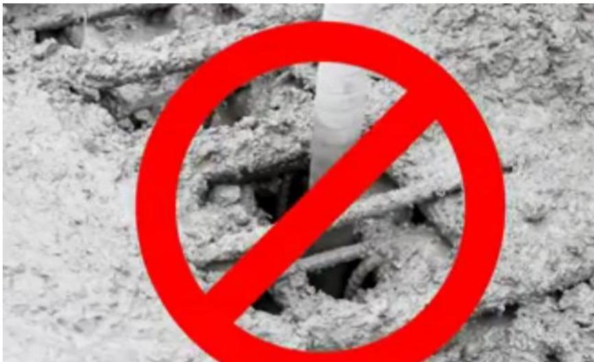
Do not vibrate longer than is necessary a few seconds per area is sufficient to liquefy the mix and remove the air.
